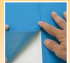
Overlapped Step Joint
