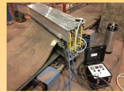
Hot Vulcanized Jointing of Rubber Belt
